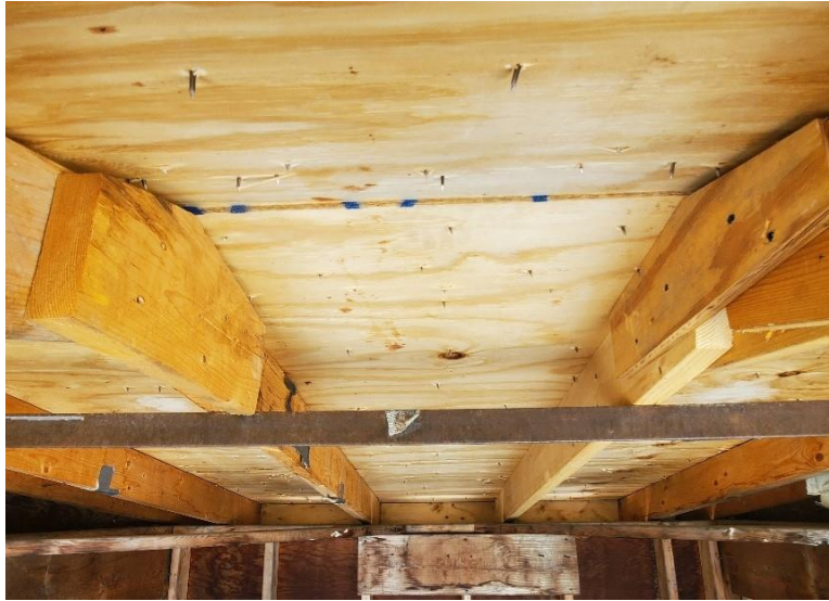
Photo No. 4 35 MPH Underside
