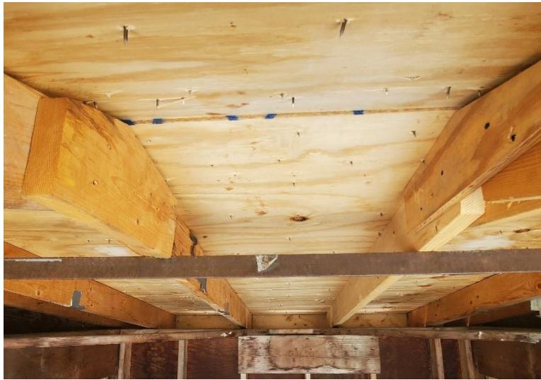
Photo No. 8 90 MPH Underside
