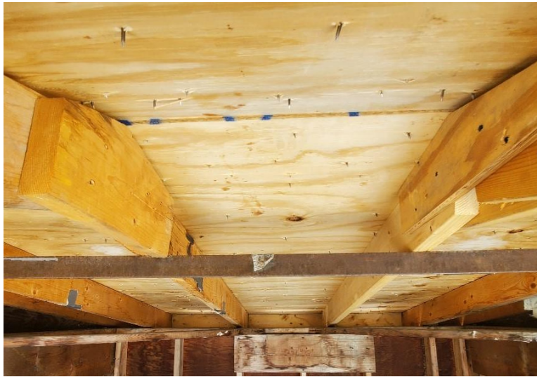
Photo No. 6 70 MPH Underside
