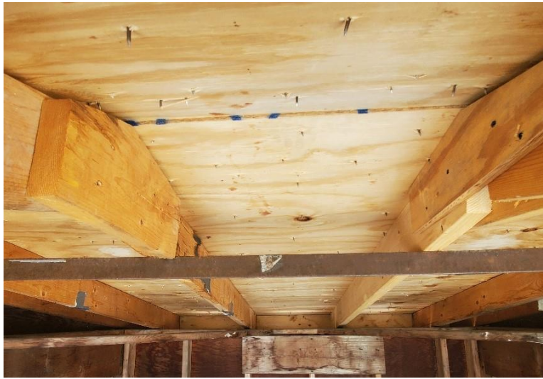
Photo No. 10 110 MPH Underside
