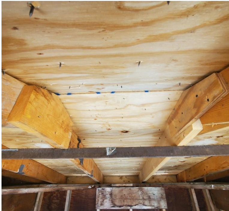
Photo No. 2 Underside Before Testing
