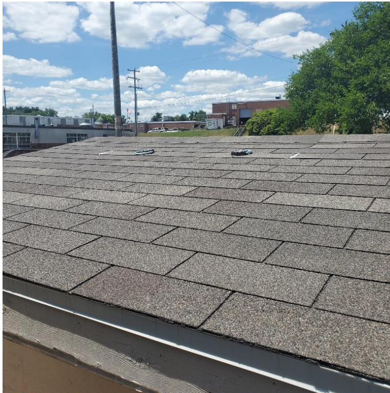
Photo No. 11 Post Test Top Side
